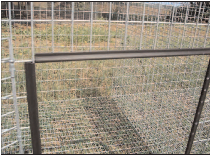
Figure 12. Cut wire showing ends covered with plastic wire guard.
